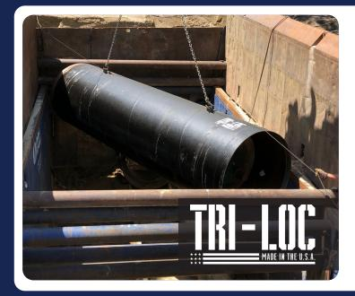
**SCOPE:** 120LF of 60" OD x .875" x 20' Tri-Loc Steel Casing - This casing was installed underneath UPRR tracks to protect a 54" carrier pipe that was needed to act as a storm sewer relief into a retention pond. Ground conditions were solid sandstone from one end to the other.
