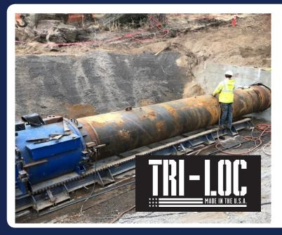
**SCOPE:** Install 330 linear feet of 42" OD x .500" steel casing pipe for a 30" gravity sewer interceptor via directional bore. The installation was on an 11% grade through solid rock at the Redmond Dry Canyon wall at the Spruce right-of-way alignment near the intersection of NW 23rd Street.
